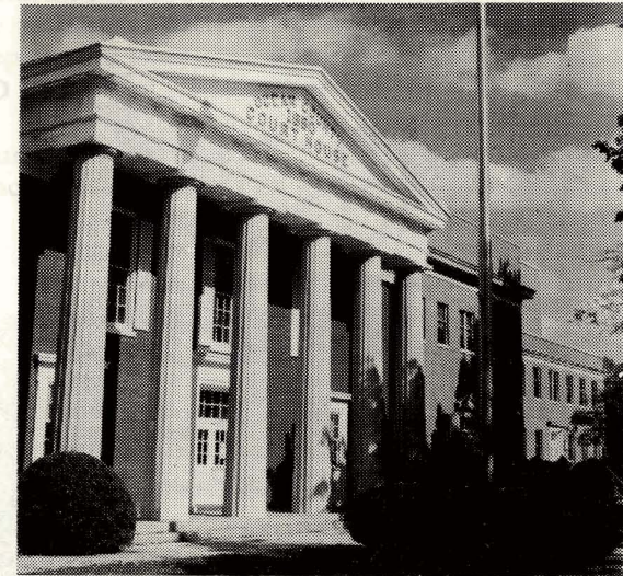
1950 East Wing Extension
